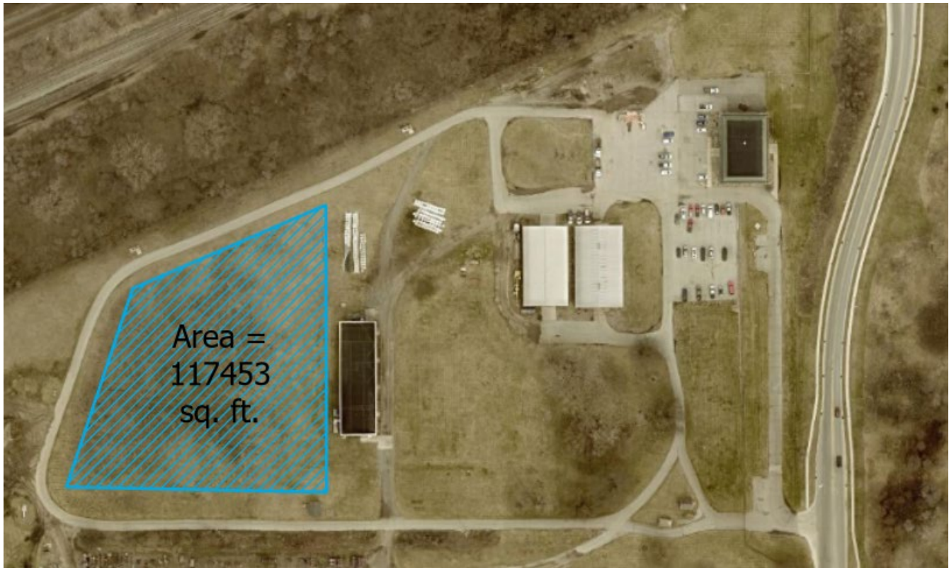
Figure 1: Olive Water Treatment Plant Available Space
