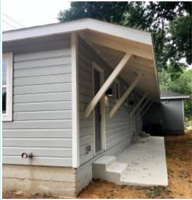
Above: Rear Entrance Walkway
