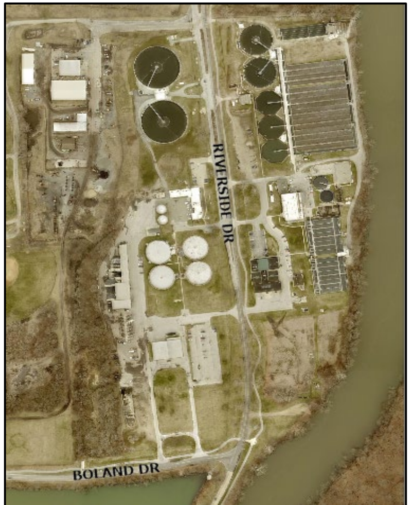
Figure 1: City of South Bend Wastewater Treatment Plant
