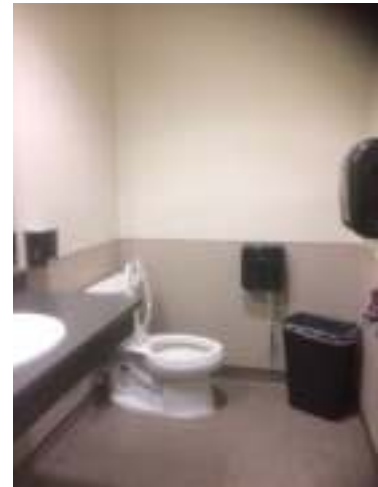
Figure 17: Example of individual washroom, 3030 Gordon
