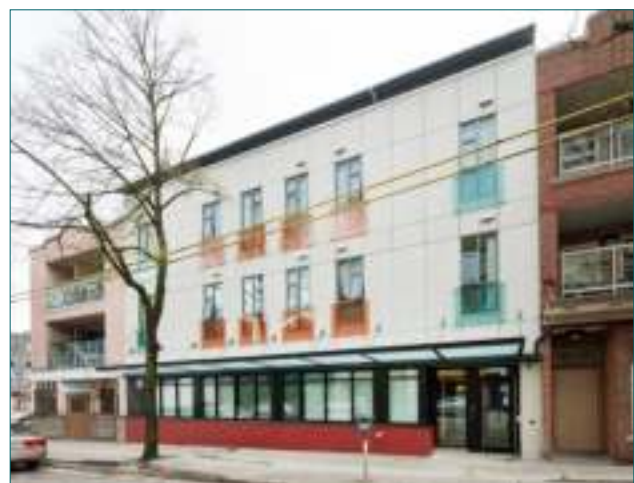
Figure 1: Powell Place, Vancouver. This 52-bed shelter involved a major renovation of an existing shelter.
