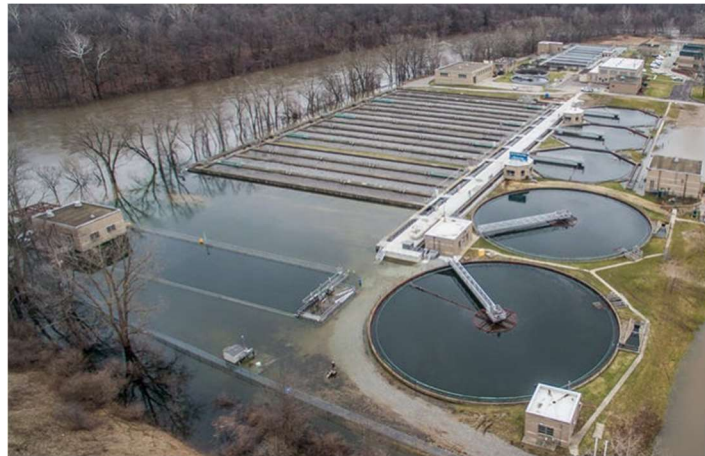
Figure A3-4. South Bend Wastewater Treatment Plant at the Peak of the 2018 Flood
