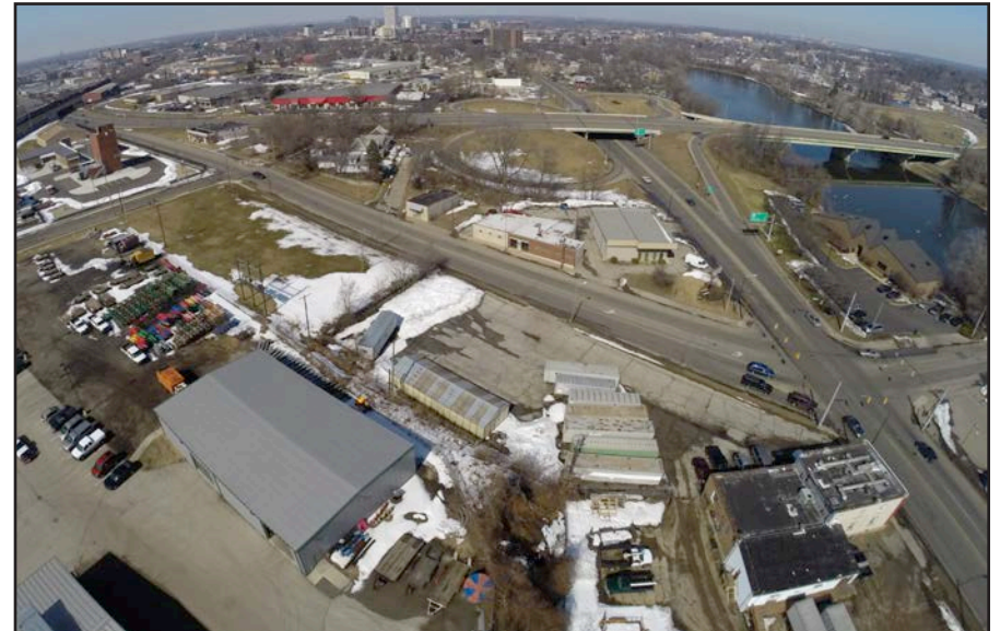
Below: Existing conditions at Lincoln Way East, Sample St. and State Road 23
