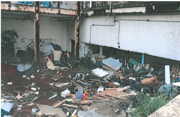
Uncontrolled Dumping at Vacant & Abandoned Building
